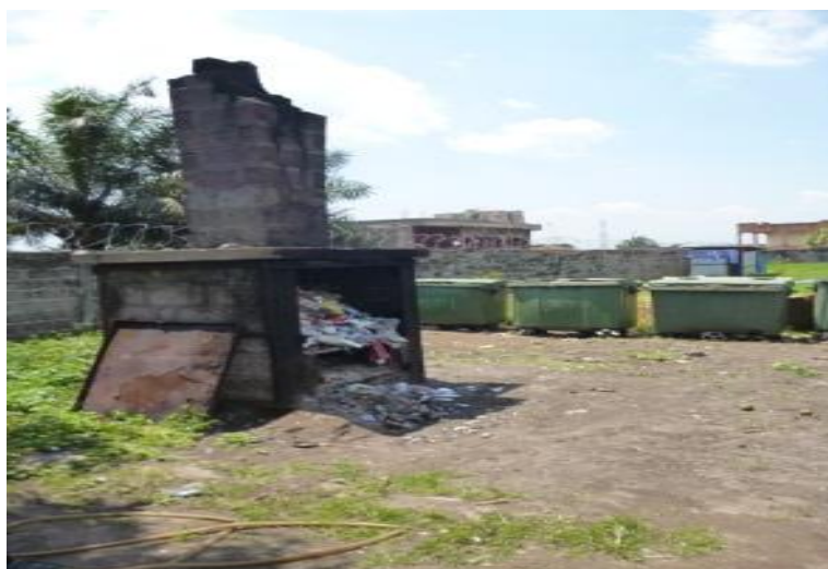
Fig. 3. Incinerator observed in a Kinshasa hospital during the survey
