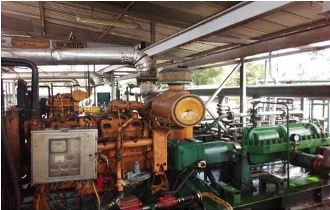
Plate 1. Gas Lift Compressor Source: Author's field work, 2020
